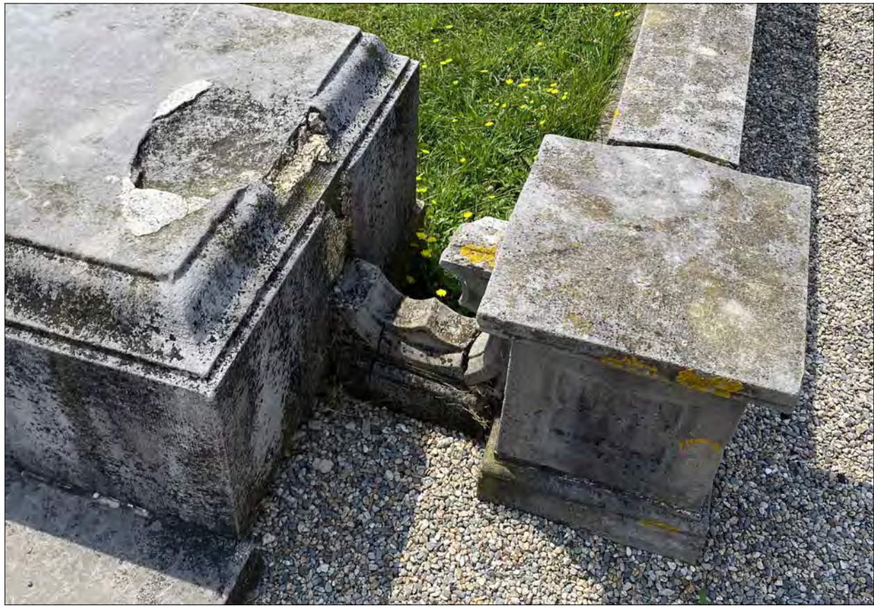
O4: EXISTING DAMAGE
