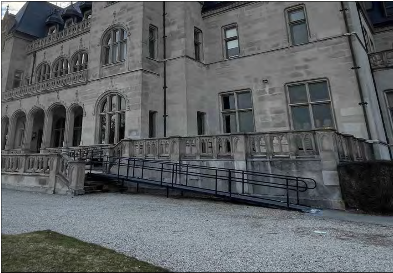
04: EXISTING OVERALL RAMPS
